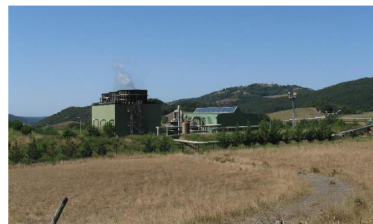
Figure 4: Le Prata (20MWe) power plant.
