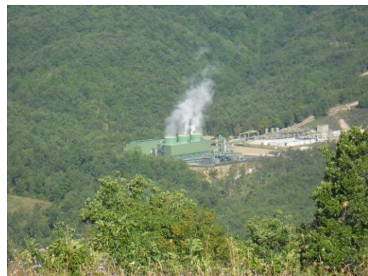
Figure 3: Chiusdino 1 (20MWe) power plant.
