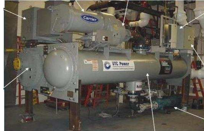
Chena, Alaska – USA, 200 kW (74 °C)
