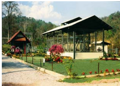
Fig. 3: Fang (Thailandia), 300 kWe
